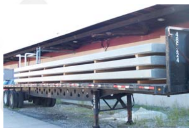
FRP bridge deck panels ready for delivery.
